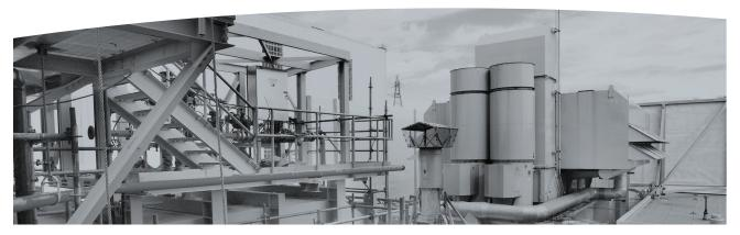
As part of NSPI's mandate for renewable energy, the Unit 6 project consisted of a 50-megawatt heat recovery steam generator to utilize waste heat recovered from two natural gas combustion turbines.
